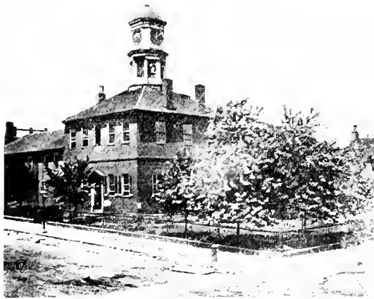
STEUDEVILLE COURT HOUSE. SERVICES 1809-1816
